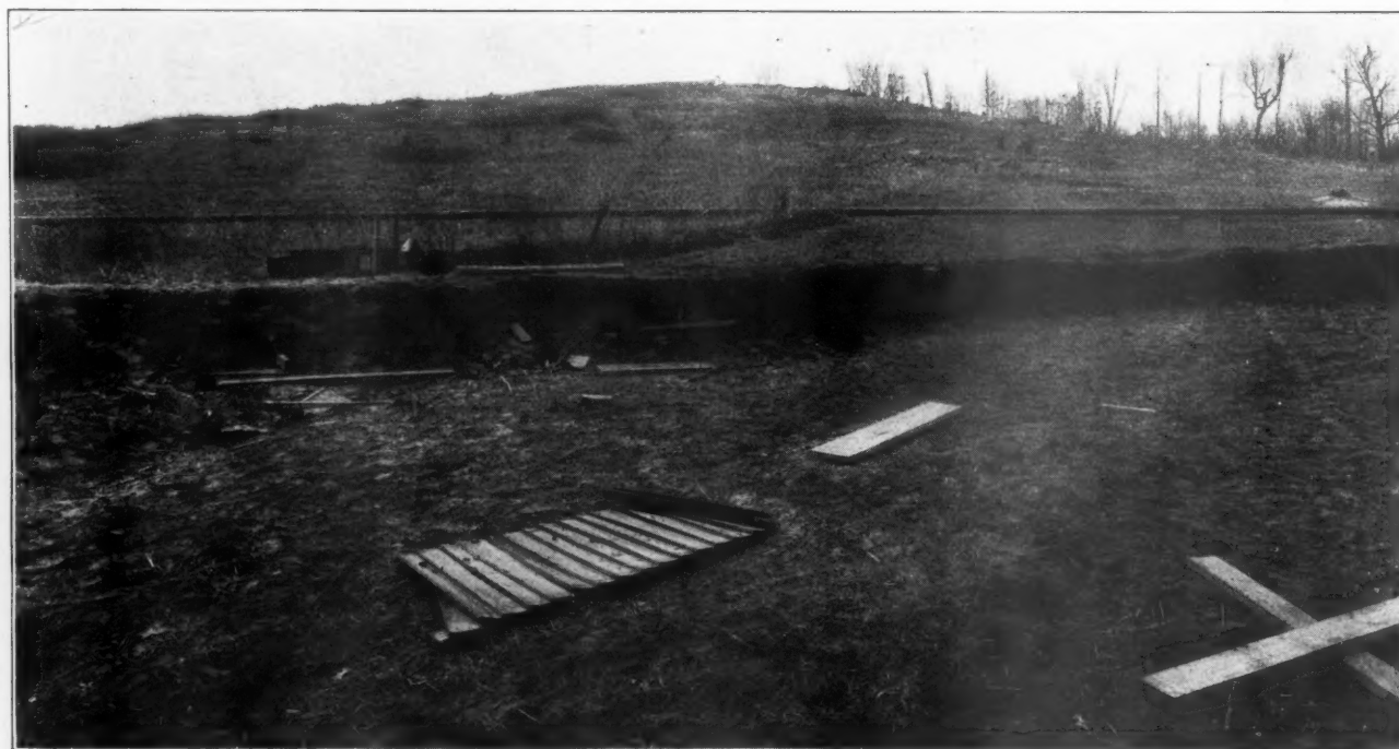
Quarry Site Before Stripping Operation
